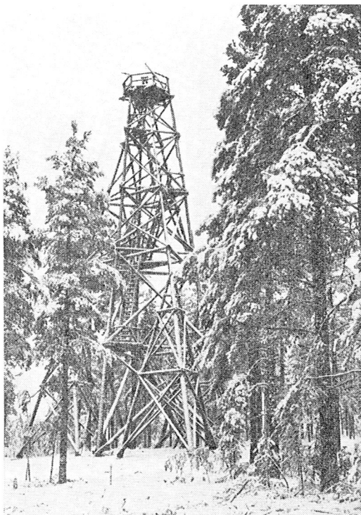
Fig. 1. The Niinisalo triangulation tower.
