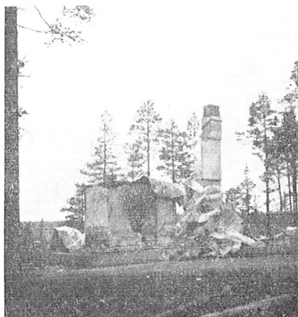
Fig. 5. Ruins of the building shown in picture 4. The higher part is the Observatory's archives vault that has been blasted.
