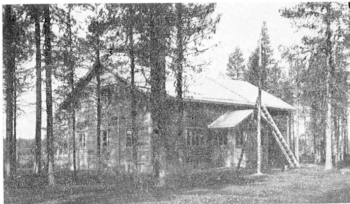
Fig. 4. Building for the Observatory staff («Morkku»).
